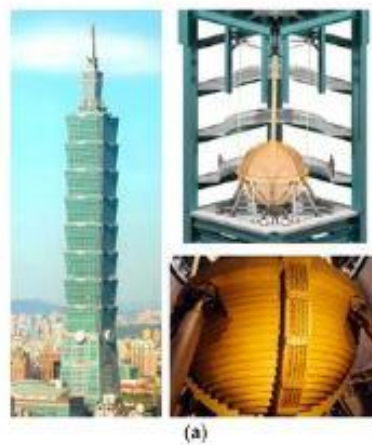
Fig 2. Taipei 101 with a sphere-shaped tuned mass damper [1]
